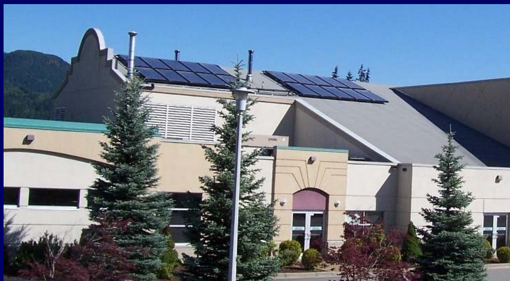
Hope & District Recreation Centre Source: Coral Engineering
