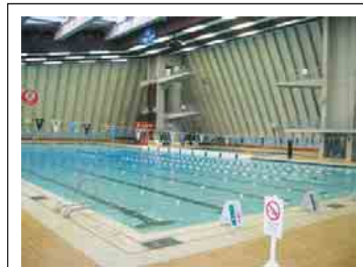
Heat recovered from natural gas-fired boilers heats the Vancouver Aquatic Centre swimming pool.
