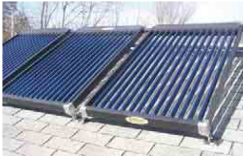
Evacuated tubes are commonly used in commercial facilities Source: Swiss Solar Tech Ltd.
