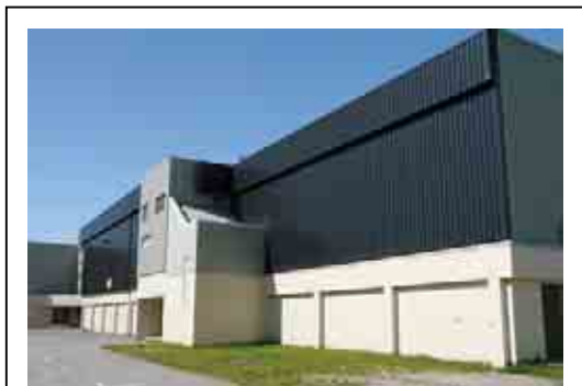
Solar wall at Seaquam Junior Secondary School in Delta, BC Source: Conserval Engineering Inc.
