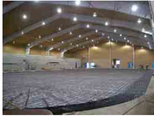
South Cariboo Recreation Centre ice rink: Ground-source loops before the concrete is poured; these loops cool the ice. Additional loops under the concrete heat the ground to prevent permafrost.
