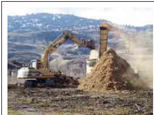
A backhoe feeds woodwaste into a chipper. This chipped biomass can be burned to generate heat and electricity.
