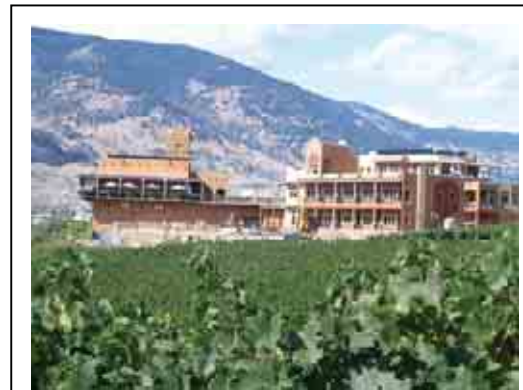
Burrowing Owl Estate Winery and Guest House, Oliver — Ground-source and solar hybrid system: 30 solar panels for domestic hot water, building heat and ground-loop support Source: Swiss Solar Tech Ltd.
